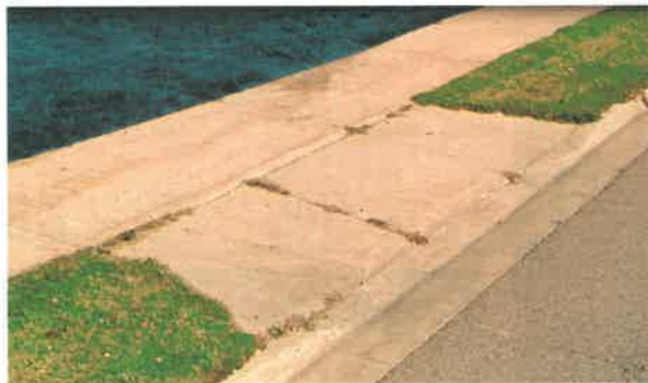
Growing grass in between concrete slabs on civic curb ramp
