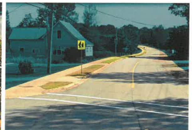
Crosswalk marking with signage on both sides
