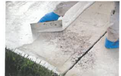
Concrete overlay/ Resurfacing
