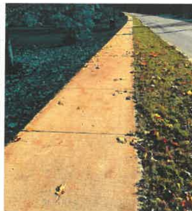
Concrete paving with even surface
