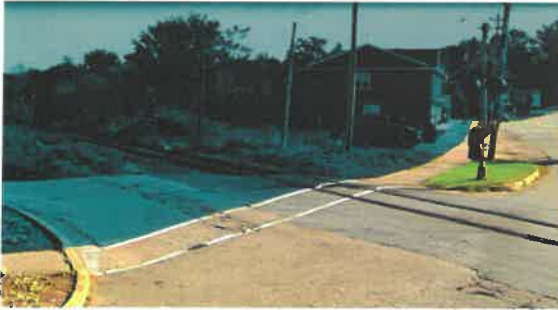
Narrow crosswalk with uneven surface
